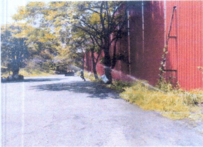
Image : Onsite Photograph of the water sprinklers in operation for suppression of dust along the raw material handling route within the premises.
