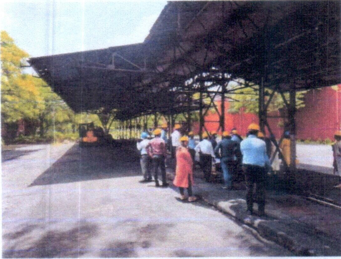
Image : photograph showing the course of physical inspection.
